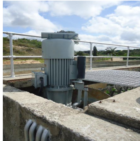
Rehabilitated sewerage systems – Addressing sanitation issues
