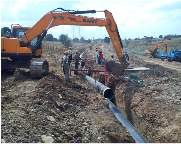
Pipeline replacement – Increasing Water
