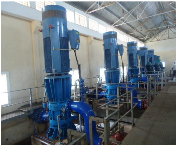
Increasing water production (newly installed pumps at the Baricho Water Treatment Plant)
